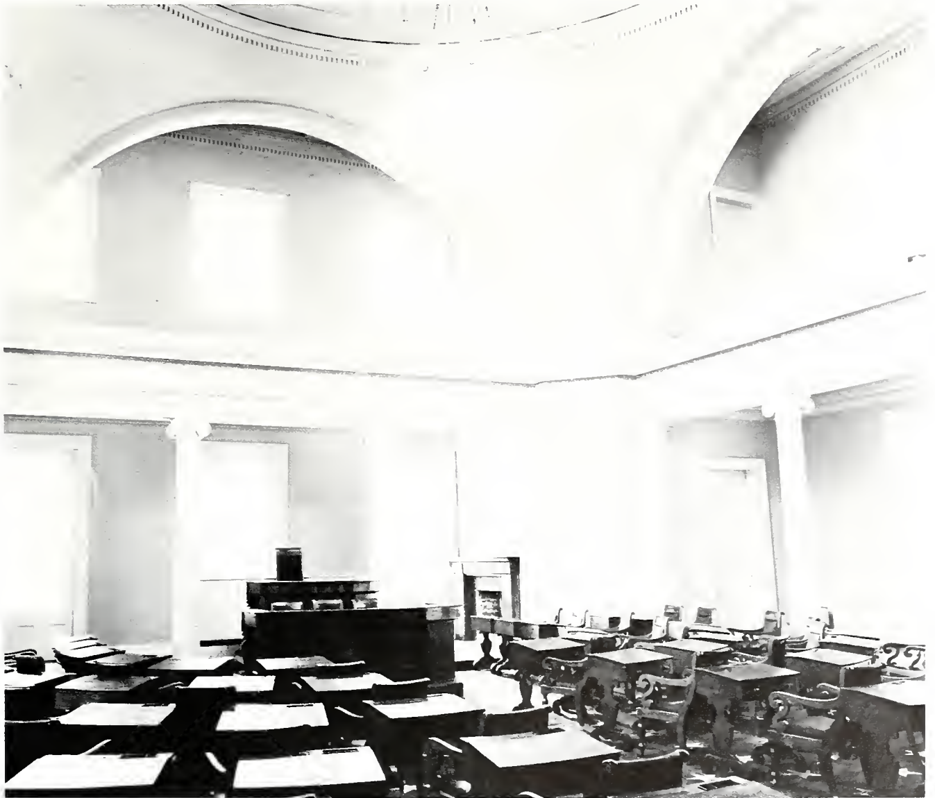
6. Senate Chamber, north wing of second floor. A shallow, circular dome covers the chamber, which is square in plan. This room was heated until 1888 by four wood-burning fireplaces, one of which is seen in the north lobby.
