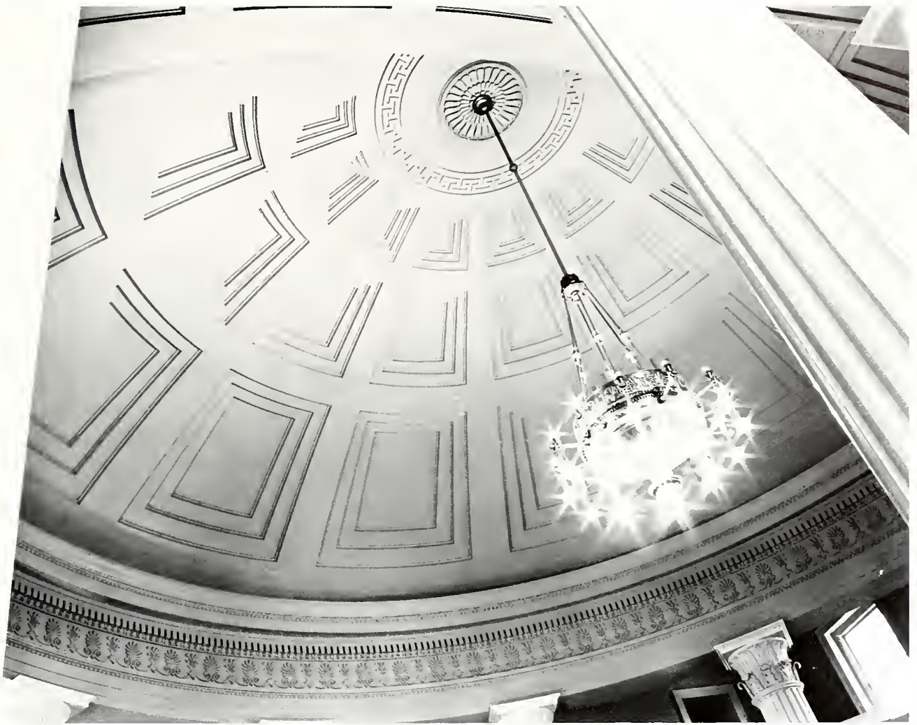
8. Detail, Fig. 7. Coffered ceiling of House Chamber. The chandelier replaces the original (1840) candle-burning chandelier and its gas-burning successor of 1866.
