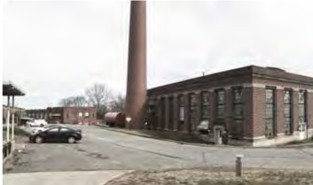
TODAY | BROUGHTON HOSPITAL STEAM PLANT
