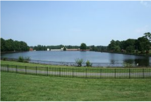
Water treatment plant, Durham, N.C. Image by Ildar Sagdejev used under GFDL version 1.2 or later .
