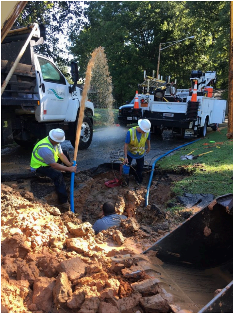
Water line repair, Gastonia, N.C.
