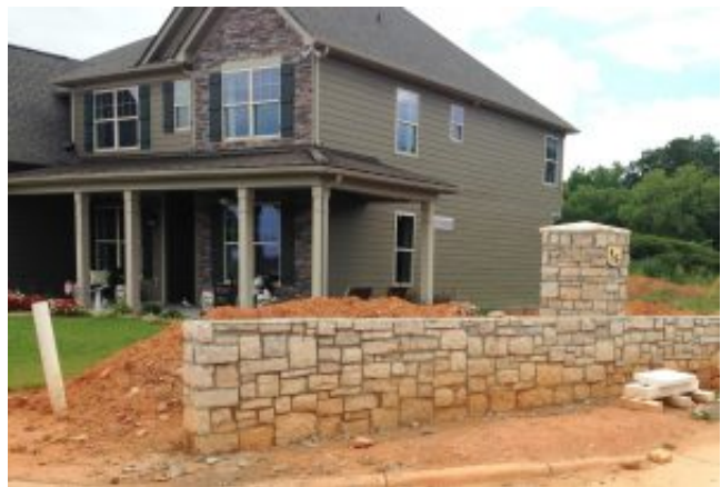
House under construction, Gastonia, N.C.
