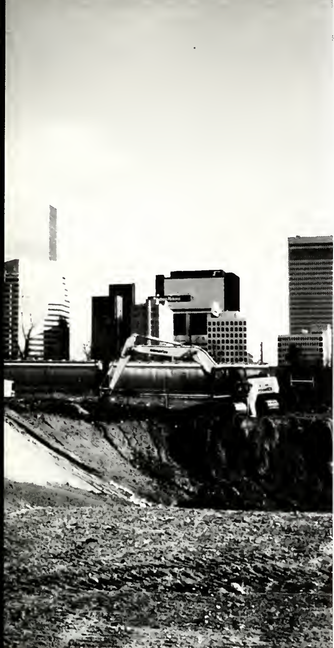
The site of the Carolina Panthers' practice facilities as cleanup began
