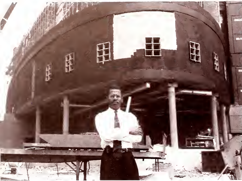
George Herron, Forsyth County Jail medical administrator, in front of the county's partially constructed $50 million detention center; it will house a state-of-the-art inmate medical facility.
