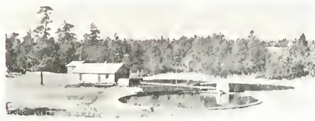
Pinehurst's modern water works and filtration plant.
