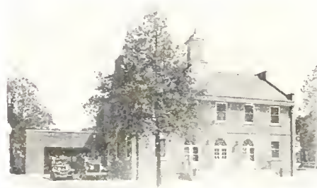
Roanoke Rapids officials recently moved into the new Municipal Building pictured above, which was constructed under the P.W.A. at a total cost of $34,000, and which gives the Halifax municipality one of the most complete and attractive city halls of any town in the State of comparable size. The new Municipal Building, which is of Georgian Colonial architecture and which is located on the main business street next to the also new Post Office, provides space not only for the city offices, court, and usual functions, but also for the police and fire departments.
