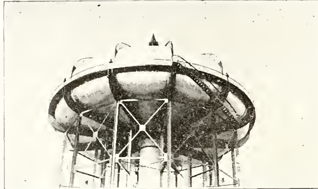
A representative project under the old PWA program—a 1,000,000-gallon tank, one unit in Rocky Mount's new water system. The pretty misses standing at the foot of the feeder pipe give some idea of the size of the tank high above.
