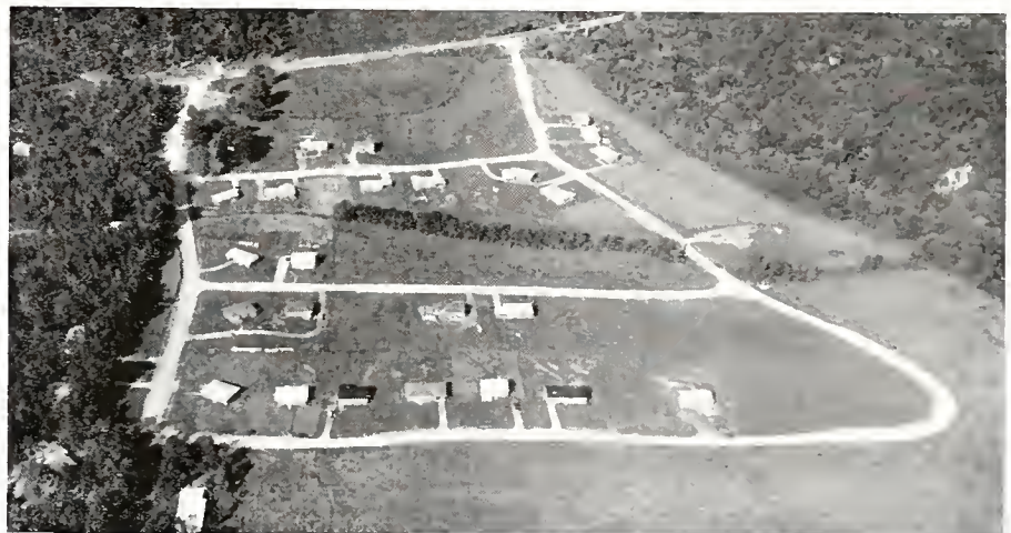
Subdivisions of the type pictured above, located some distance from a city, often have need for water and sewer services and may request aid from the county in providing these services.
