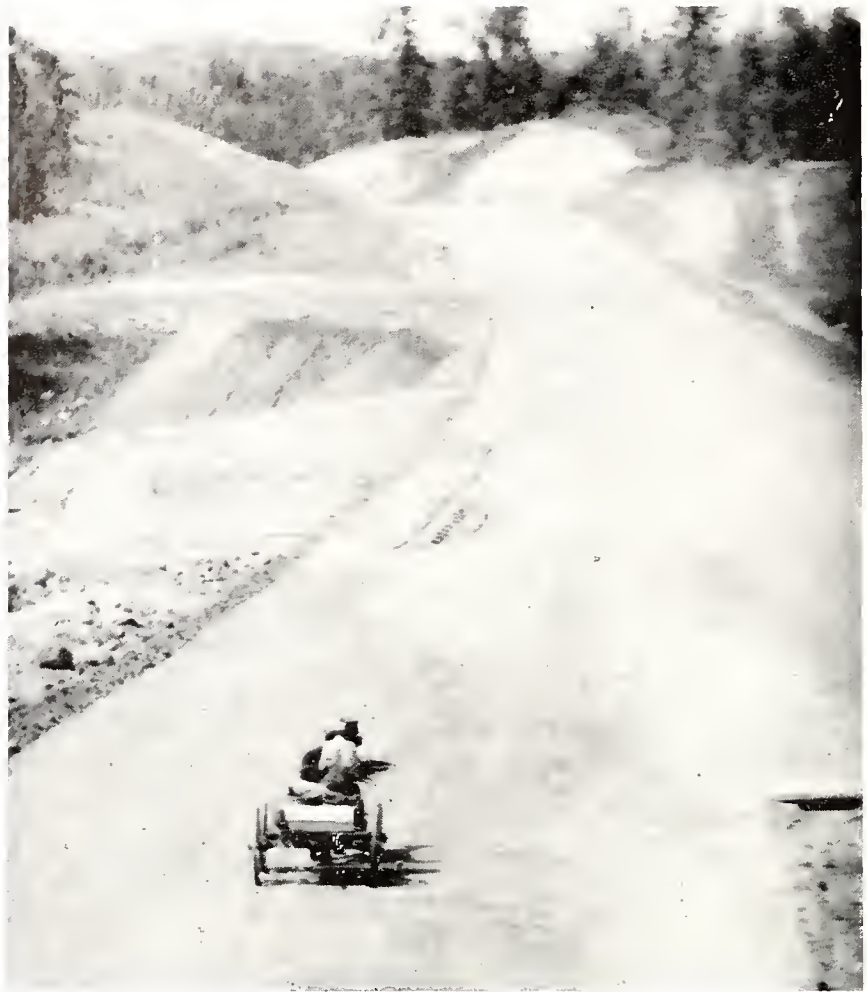
Beginning of a new era in highway transportation
