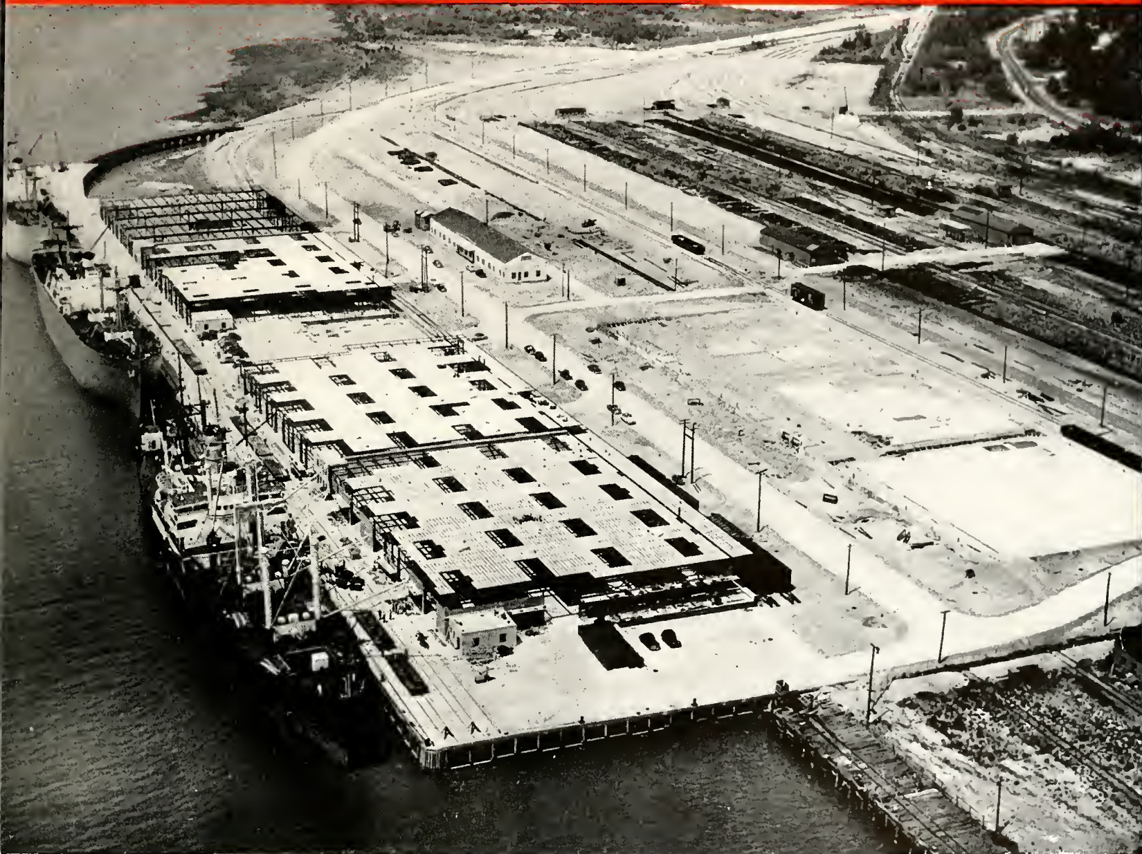
The Wilmington Port Terminal
