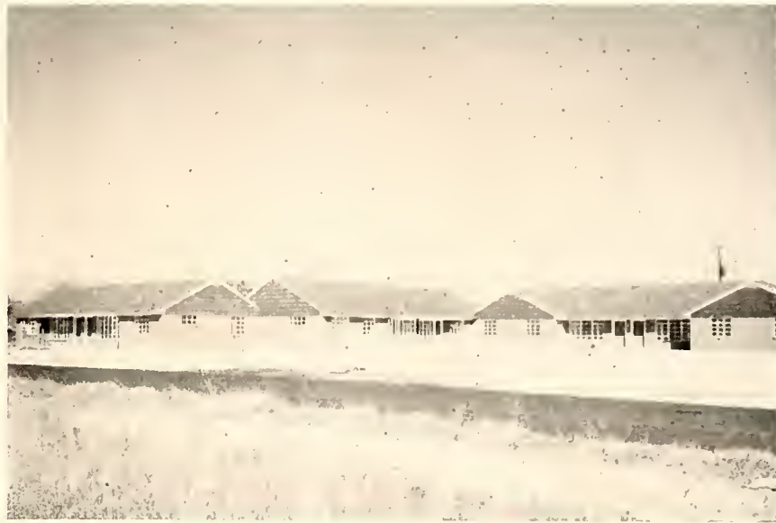
This unit (in Goldsboro) is typical of housing being built for needy tenants all over North Carolina.
