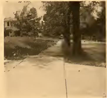
by tree roots. Result: costly maintenance, possible damage suits by persons injured through failure to maintain sidewalk in safe condition.
