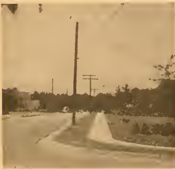
operation of property owners will be necessary for such a plan, but the advantages offered—safety and convenience, easier maintenance and a better chance for permanence—seem to make it worth the effort.
